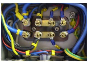
AC CONNECTION BOX SHOWING TERMINAL CONNECTIONS
